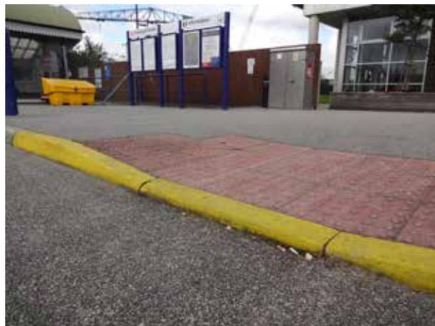
*This dropped kerb, on an accessible route from parking to station entrance, is appropriate in principle, but is not flush and will present an obstacle to some users.*
