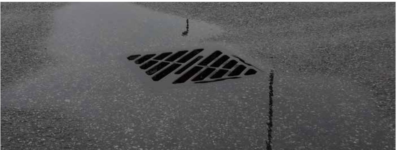
*Ponding can be an inconvenience or even a danger for customers. In this example, minor ponding appears to be a result of mismatched surface levels. In other cases, it is an indicator of blocked gullies or drains.*
