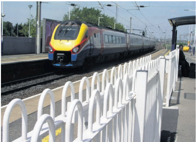
Fencing on some stations now shields the fast line platforms, helping to discourage someone in distress from accessing them
