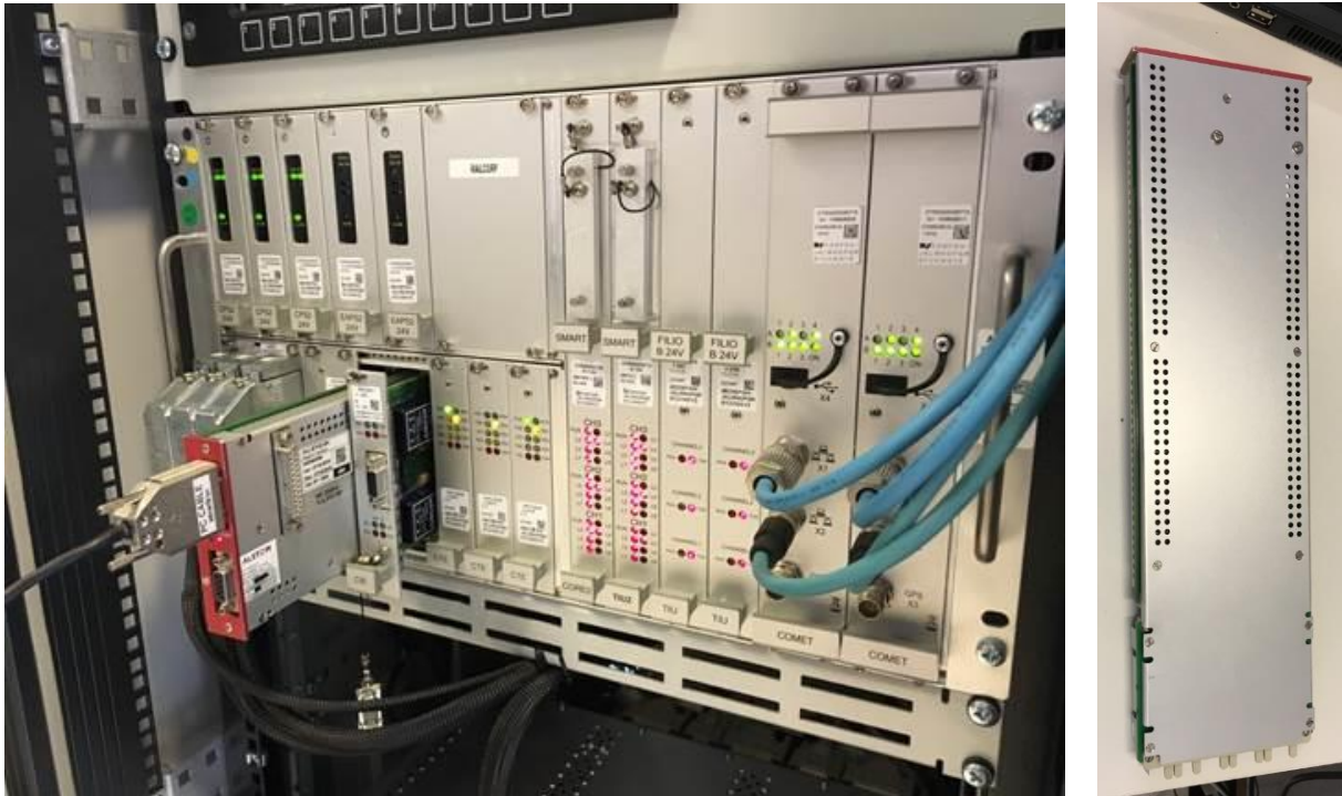
Figure 4: Laptop connected via maintenance card, and the card shown to the right
