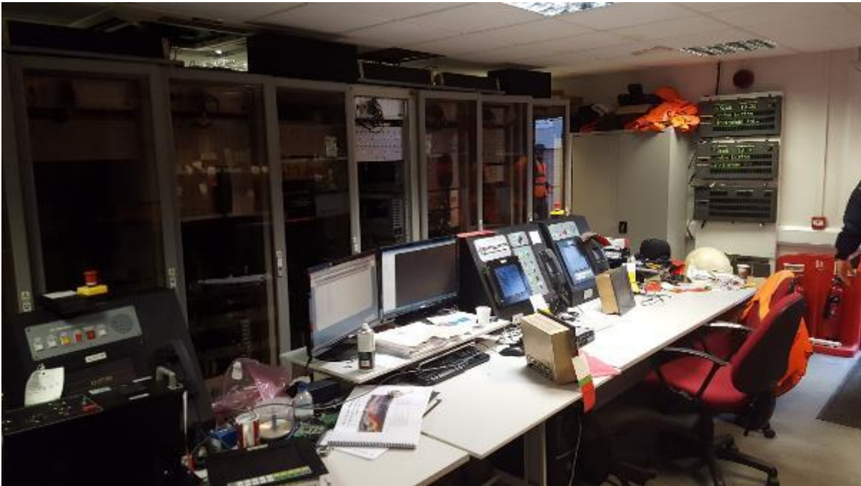
Figure 8.1: Alstom's TMS simulator at Oxley Depot
