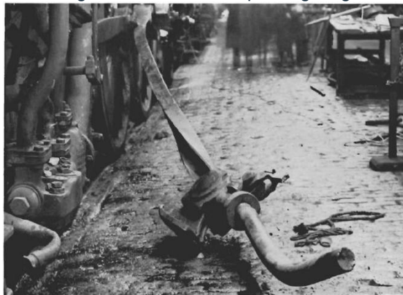
Photograph 1. The Britannia locomotive showing the displaced motion assembly.
