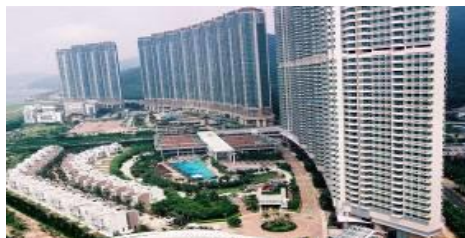
Tung Chung Station Development
